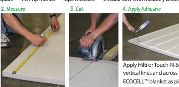
Start at a square corner of the room. Measure length and width of blanket needed saw equipped with a for wall application. Then measure and mark blanket.
